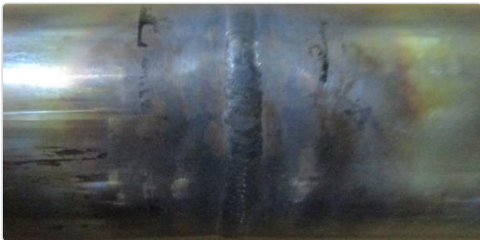
Cupronickel weld before
