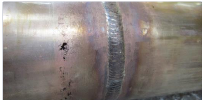
Cupronickel weld after
