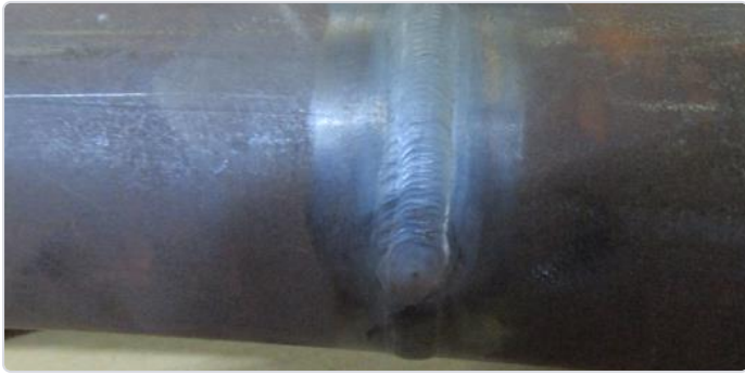
Mild steel weld before
